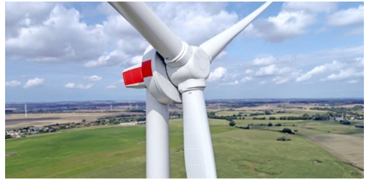
HYGRO specialises in the production, delivery and distribution of hydrogen produced directly from wind. It is building a 4-MW wind turbine with an integrated electrolyser in the province of North Holland. The aim is to maximise synergy between wind power, hydrogen and pipeline & storage technology. The concept optimises conversion of wind power to hydrogen, which can be transported at much lower cost than electricity and with a significantly lower impact on spatial planning.
